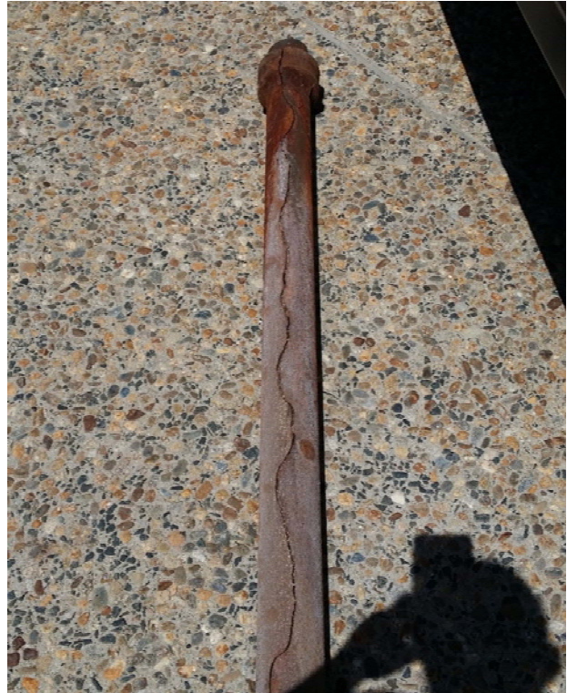
Cracked drain removed for repairs in Spring 2018
