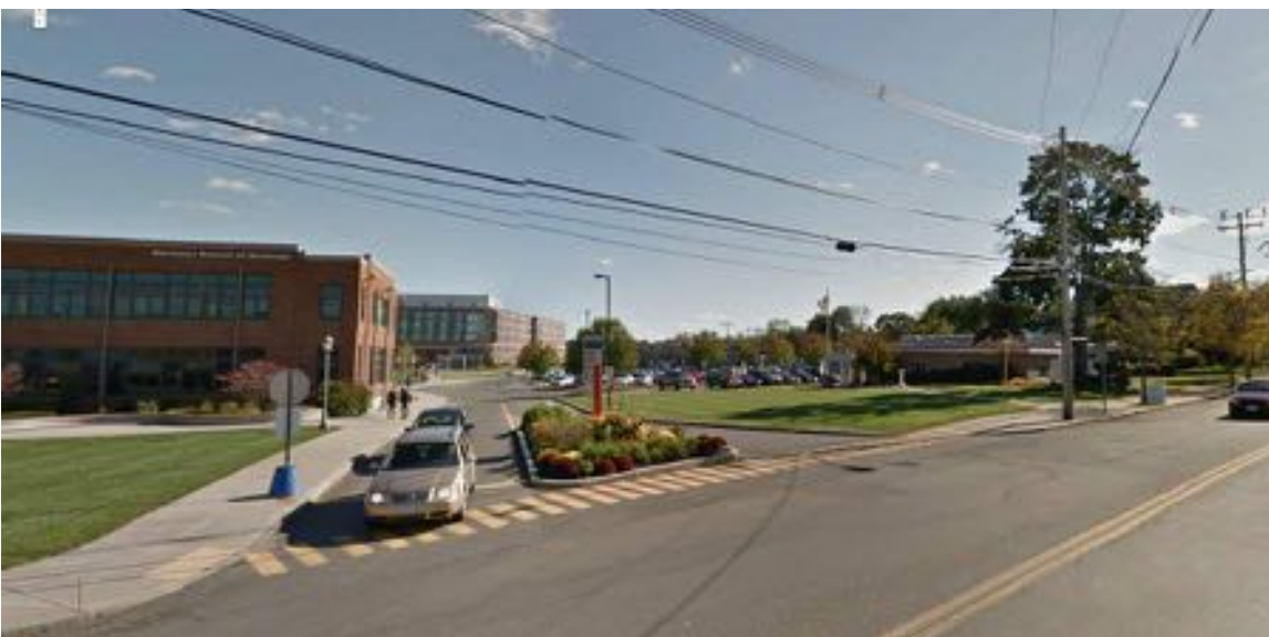
EXISTING ENTRY TO CENTRAL CAMPUS OFF OF LORING AVENUE, WITH THE SCHOOL OF BUSINESS AT LEFT AND CAMPUS POLICE AT RIGHT.
