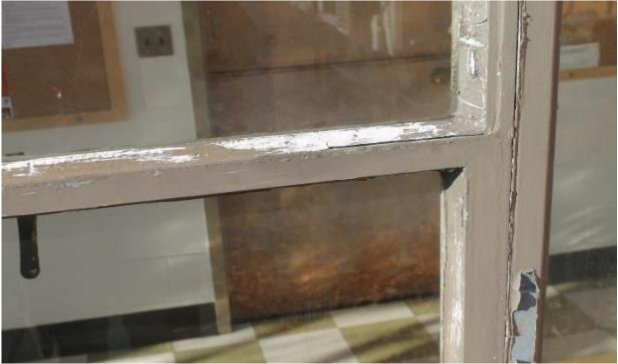
Photo 9: Brown and white window caulk on Boiler Plant roof
