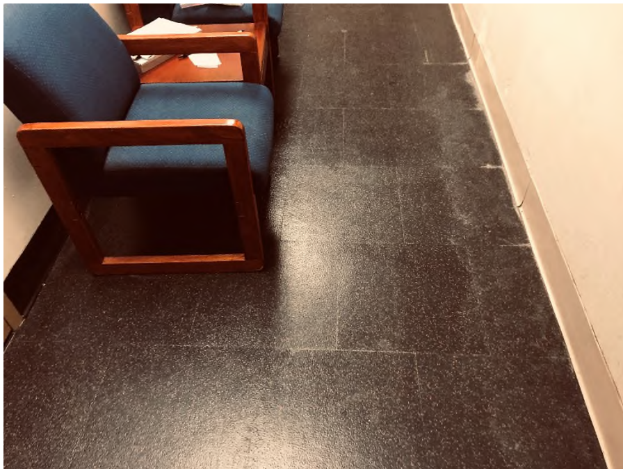
Black with red speck floor tile/mastic, black and white cove base and mastic in Adjoining Corridor
