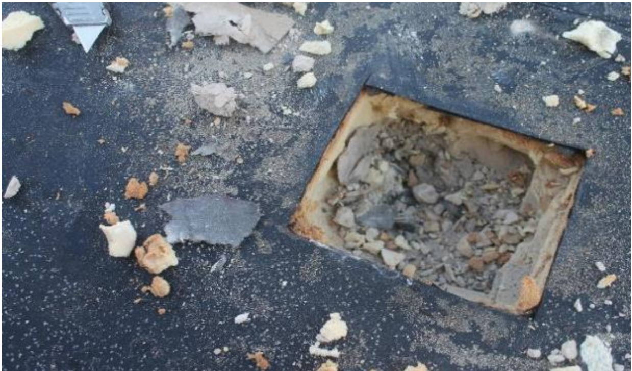
Photo 4: Rubber membrane, Styrene, black paper and DenDeck on concrete Connector roof
