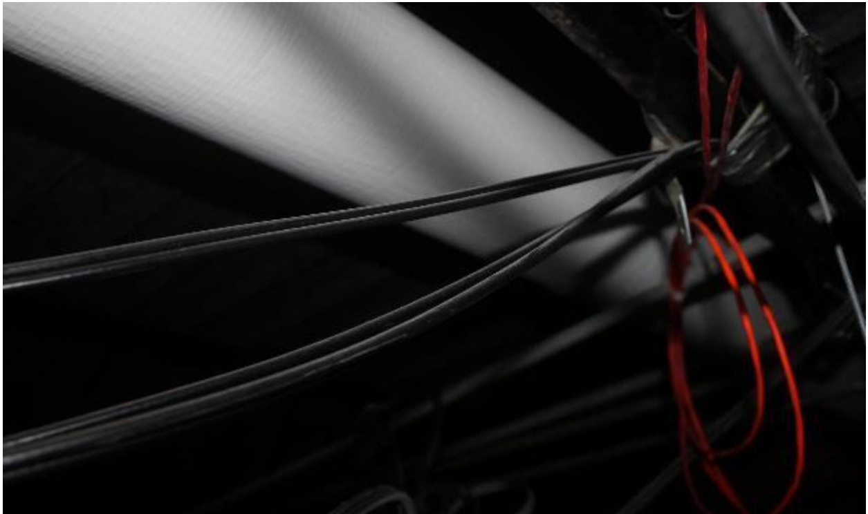
Photo 12: Fiberglass insulation on crossover roof drains
