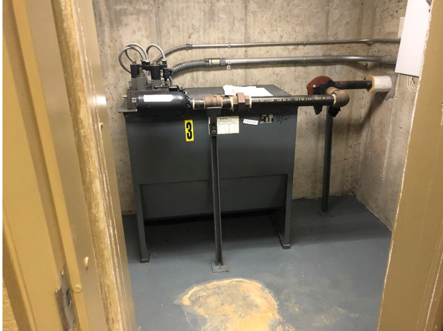
Elevator machine room
