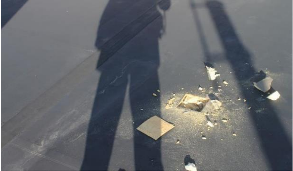
Photo 5: Rubber membrane, Styrene, black paper, and DensDeck on concrete Administration roof
