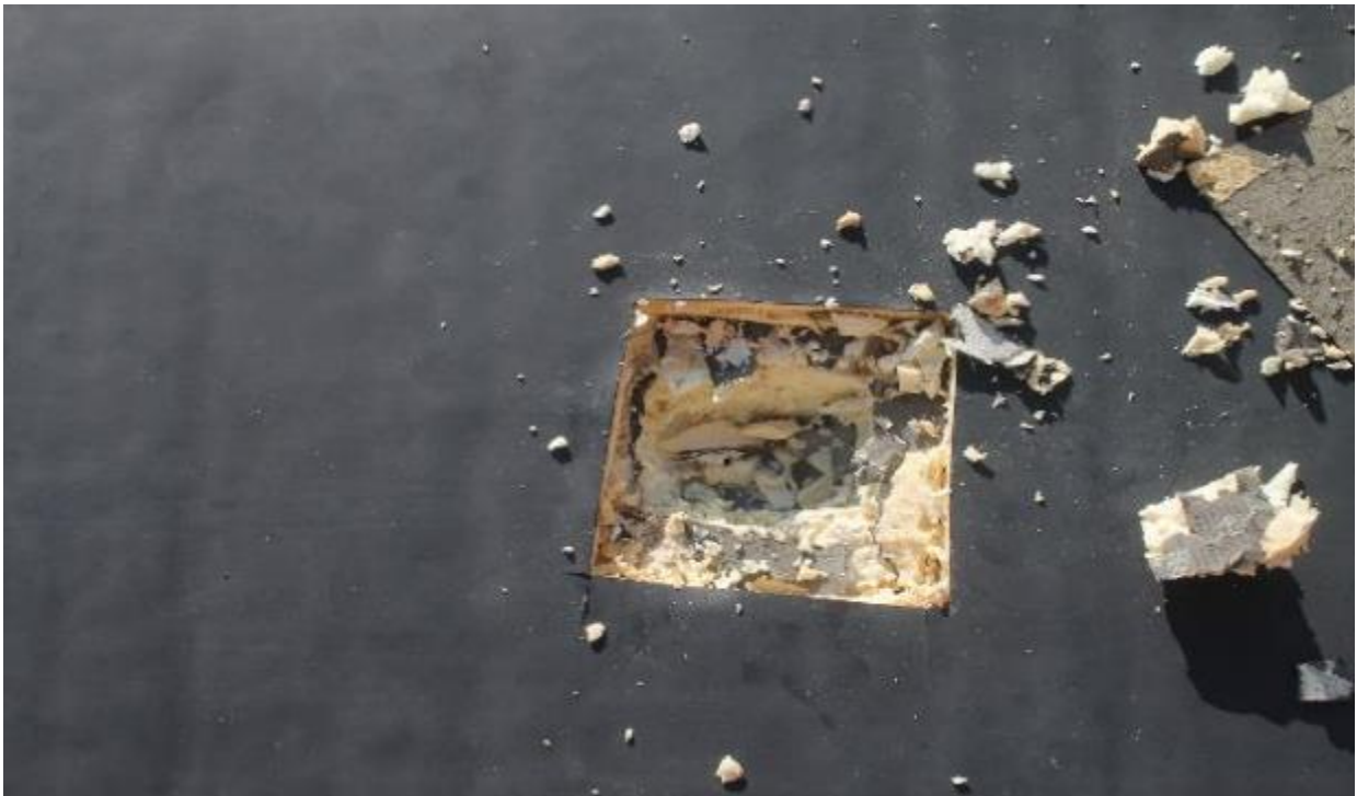
Photo 8: Rubber membrane, Styrene, and black paper on concrete Boiler Plant roof
