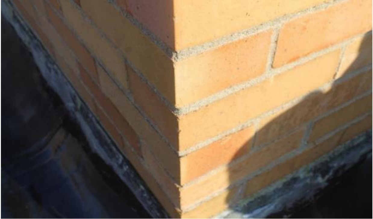
Photo 7: Black flashing mastic on brick wall on Administration roof
