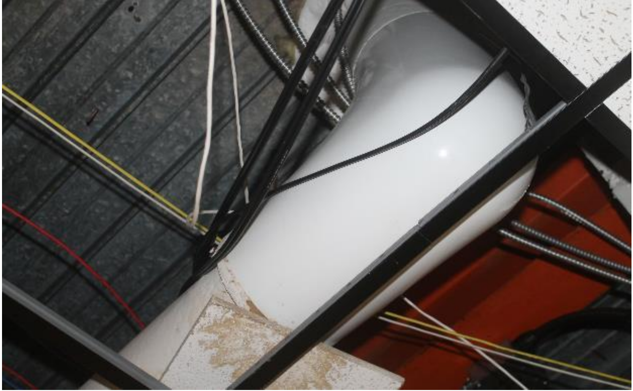
Photo 15: Fiberglass insulation on Administration building roof drains
