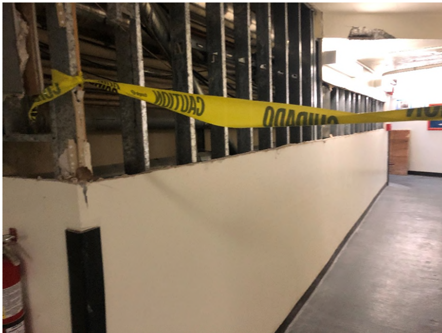
Gypsum wallboard and associated joint compound in the Main Corridor
